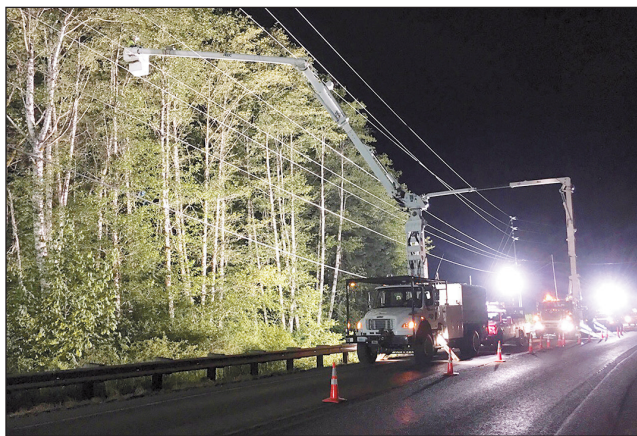
Vegetation Department and Line Crew performing nighttime tree trimming along Hwy 112 in order to not block traffic during the day.
