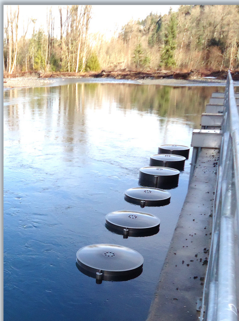
Elwha Surface Water Intake Screens
